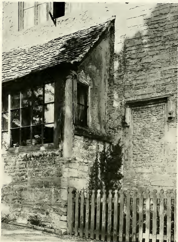
DETAIL OF OLD HOUSE AT BURFORD
